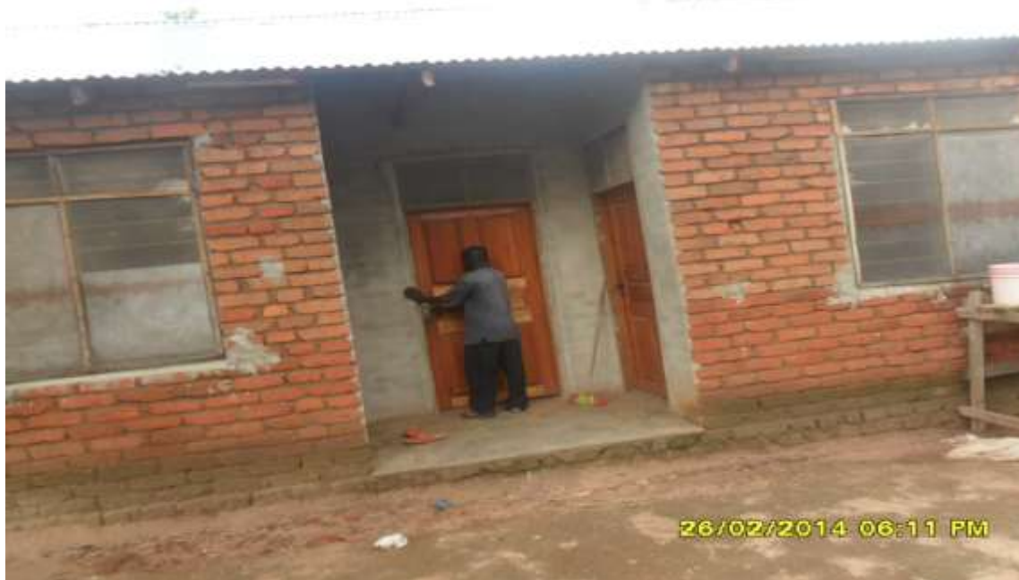
Chicken House with three partitions constructed
