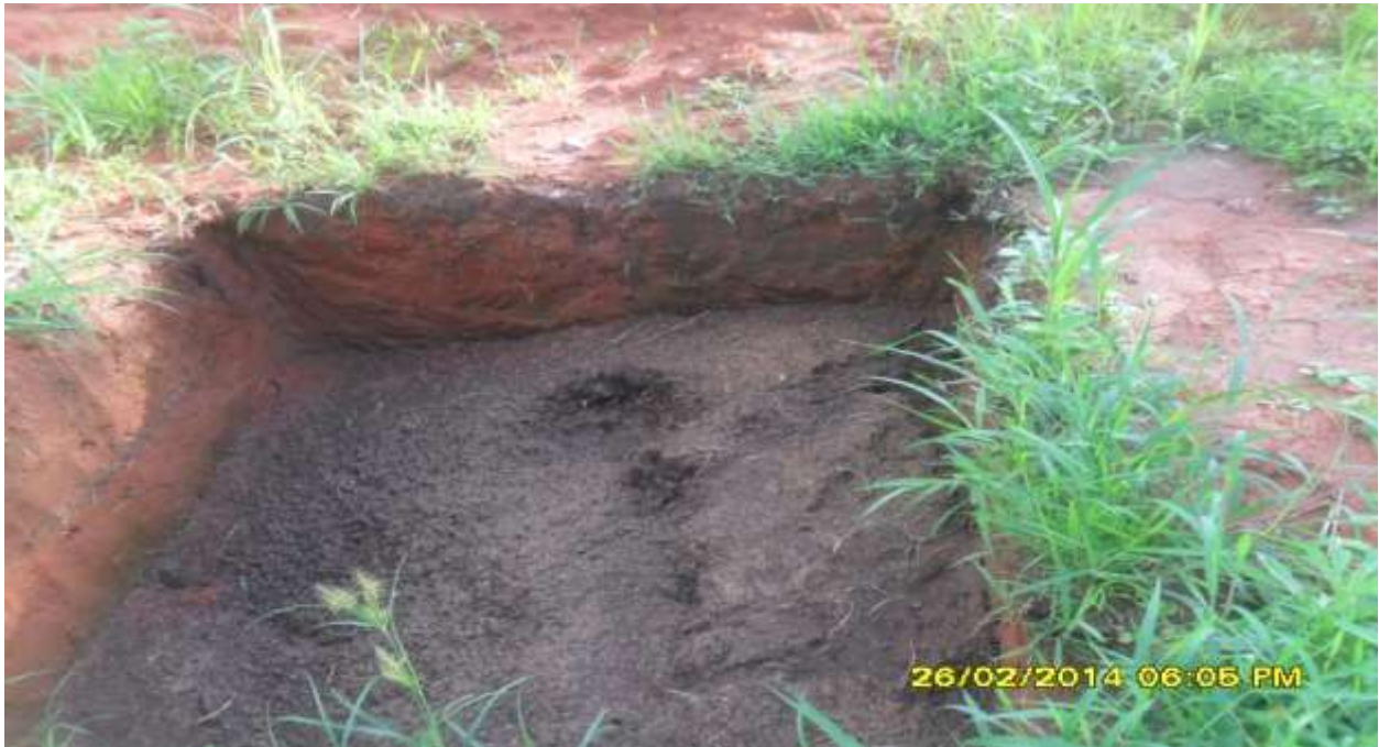
Manure pit constructed
