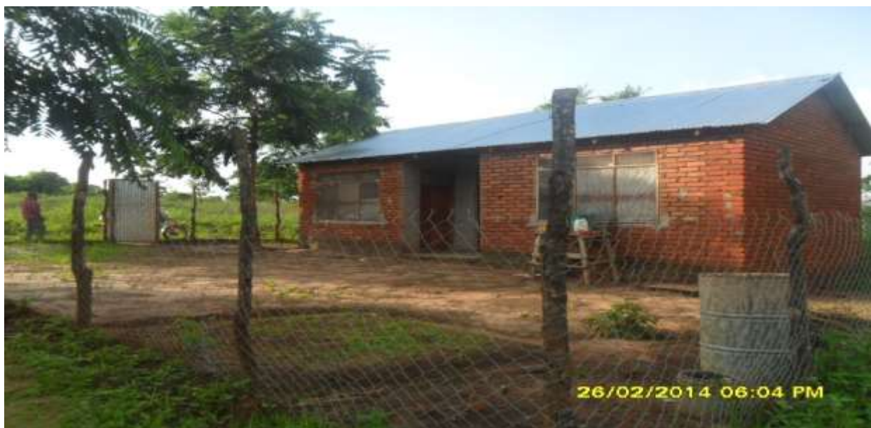
Iron Fence constructed
